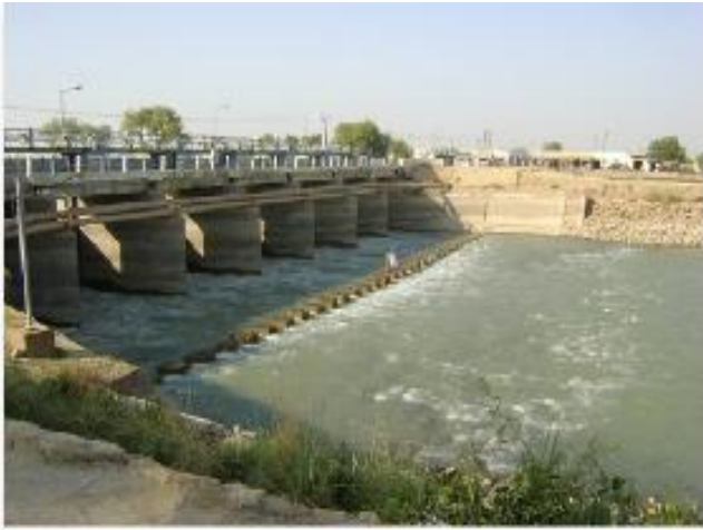
Figure 1. The Head Regulator of the Phuleli Canal
